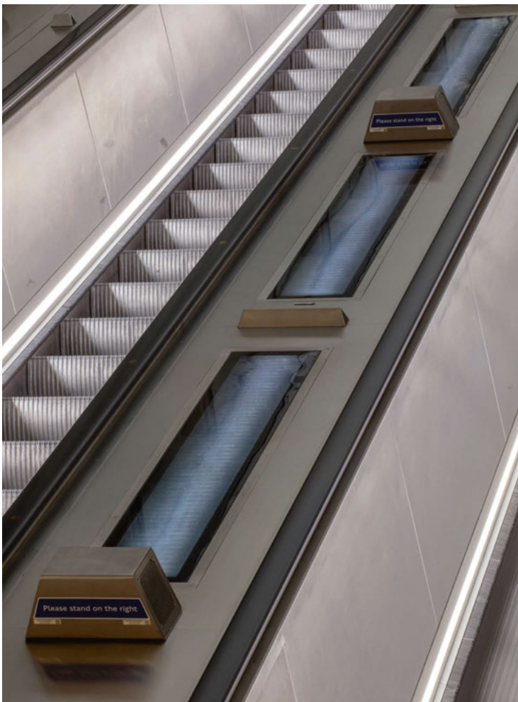
On the escalator tunnels leading to the station platforms, Future Designs' Plinth luminaires recessed into the elevator deck create an elevated feel, while custom filters within the fixtures eliminate glare.
